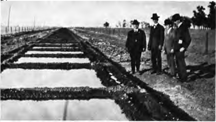
Inspecting method of ponding concrete roads. Left to right—Senator Moser of Oregon. Division Engineer Caruthers, Office Engineer Dodge, G. Cameron Parker, Dominion of Canada Department of Highways.
